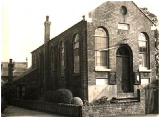
Zion Chapel Trinity Lane Hinckley demolished 1988
